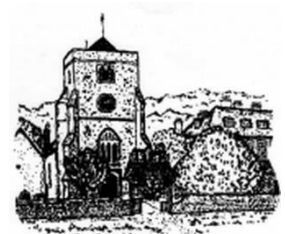
St Botolph's, Bradenham
